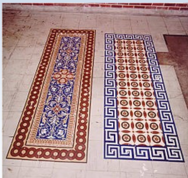
Encaustic clay tiles produced by the Maws Company in the 1800s. The coloured clay goes right through the tile so it stays the same as it wears down from use.
